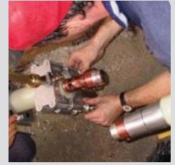
ON-SITE CABLE END PREPARATION
