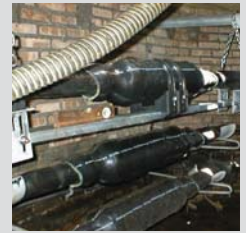
COMPLETE JOINTS IN FINAL POSITION
