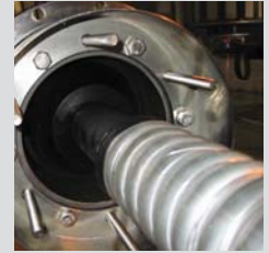
STRESS CONE POSITIONING
